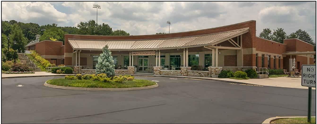
Watershed Building at Cedar Springs Presbyterian Church, Knoxville. Copyright Ron Sentell.
